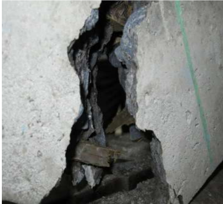
Fig.13: Failure of Doubly Reinforced Beam
